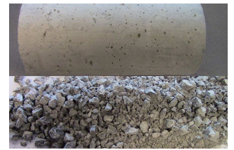
ciment drill core
